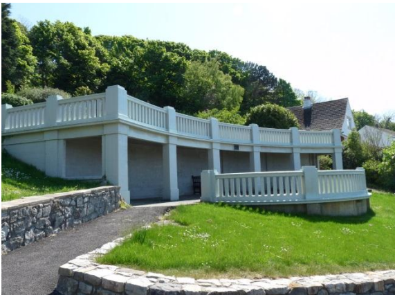
Hillside Shelter, Prestatyn – a Grade II listed 20 th century structure, listed as an unusual and innovative concrete garden structure, the centrepiece of a public garden
